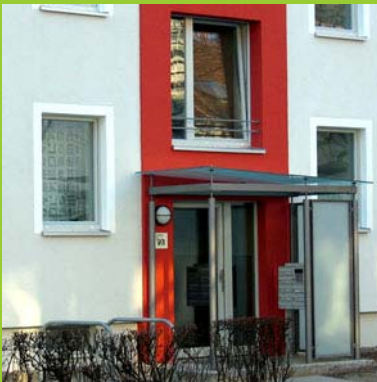
picture 3.3 – refurbishment; Source: architectural office pk nord
