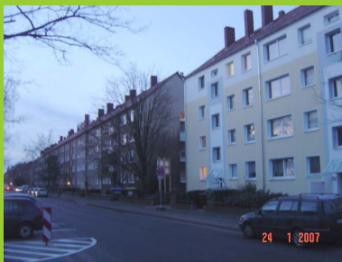
pictures 4.3 and 4.4 – on-site session, here: thermo graphic portrayal after refurbishment; Source: GMW – engineering office GmbH
