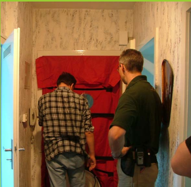
picture 4.2 — on-site session, here: Blower door test; Source: GMW engineering office GmbH
