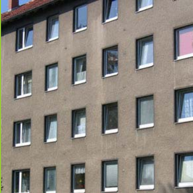
picture 3.1 – current facade; Source: architectural office pk nord
