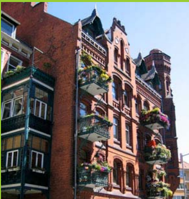
picture 3.2 – current facade; Source: architectural office pk nord
