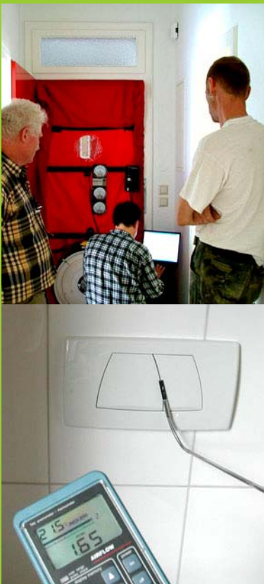
pictures 5.3 and 5.4 – 2nd meeting; Blower-Door is installed. on the bottom: Anemometer in use Source: GMW – engineering office GmbH
